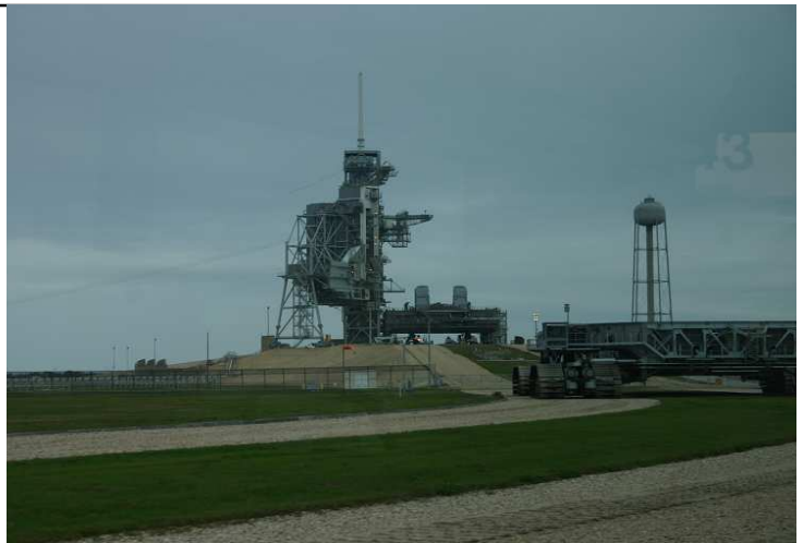
Pad 39-A with the crawler transporter in the foreground
